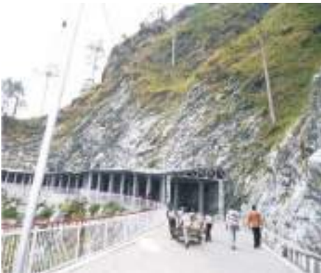
Fig. 7.39: Tin Roof sheds to prevent direct impact of rock fall
