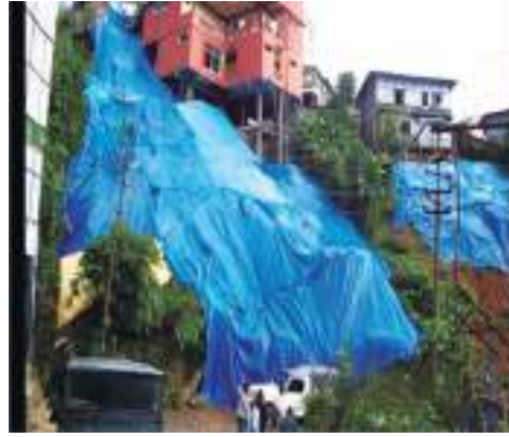
Fig. 1.45: Residents protect houses by using polythene sheets to prevent seepage
