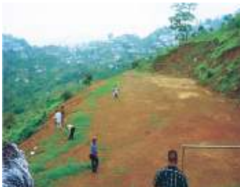
Fig. 1.30: Ground cracks indicating incipient slope failures
