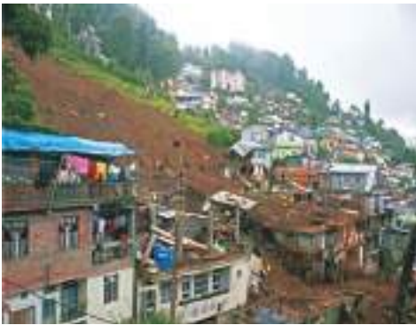
Fig. 1.52: Landslide affects cluster of houses at foothill slopes
