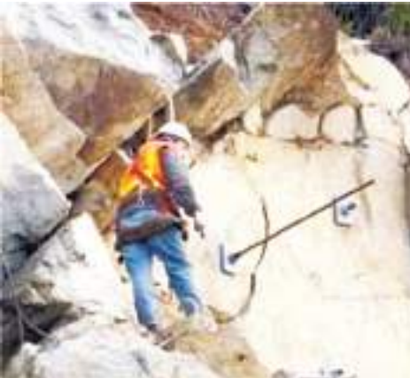
Fig. 7.57: Rock Bolting
