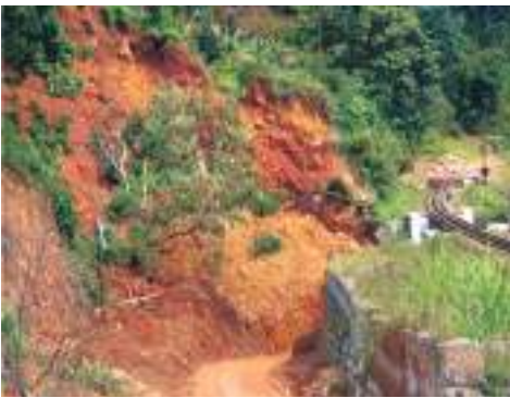
Fig. 1.54: Landslide causes damage to railway track and road
