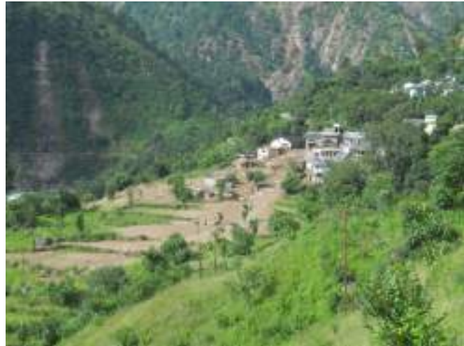
Fig. 30. Photograph showing debris flow around Chunni village.
