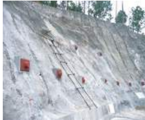
Fig. 7.34: Rock bolting and shot creting for slope stabilization
