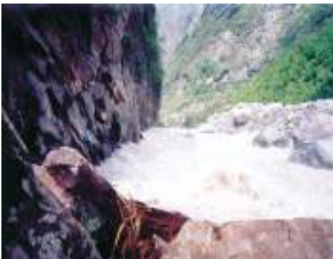
Fig. 1.48: Complete road washed off after bursting of transient landslide dam
