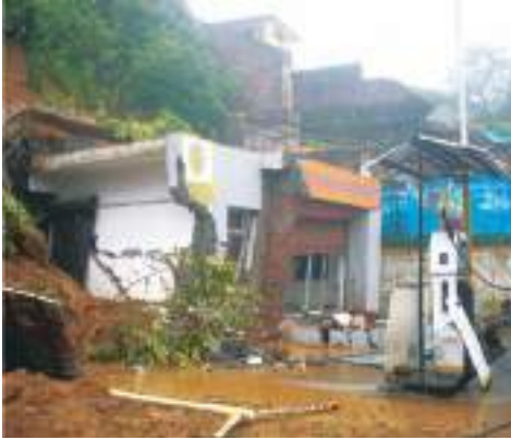
Fig. 1.50: Petrol pump damaged leading to fuel shortage
