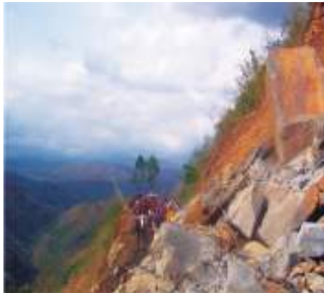
Fig. 7.58: Rockfall blocking road
