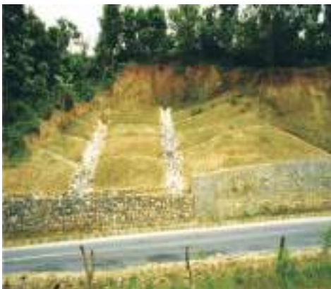
Fig. 7.53: French drains
