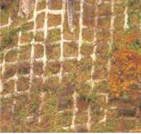
Fig. 7.1: Spraying crib works for preventing surficial failures
