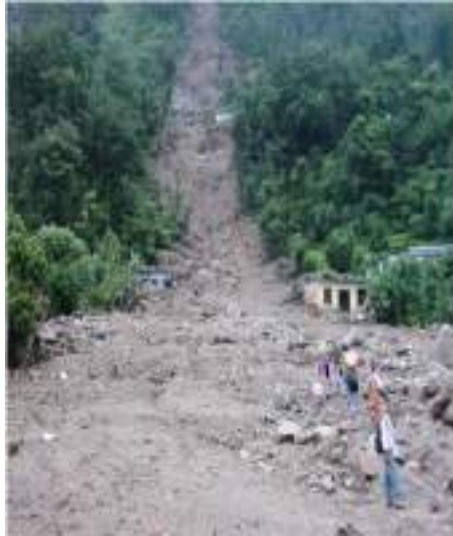
Fig. 31. Photograph showing devastation caused by debris flow around Mangoli.
