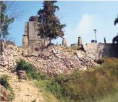
Fig. 1.56: Heritage building at risk from landslides
