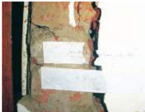
Fig. 1.35: Monitoring wall cracks using paper slips with markings
