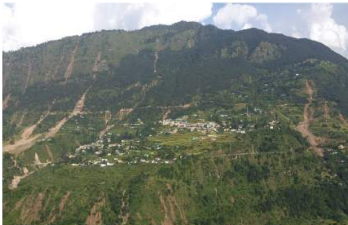
Fig. 2. Panoramic view of Okhimath town showing scars made by the debris descending down the steep slope.
