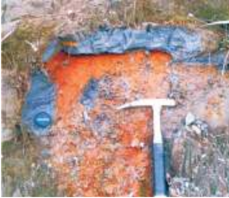
Fig. 1.26: Seepage and leaching at junction between sand & clay beds
