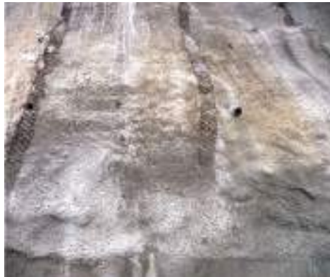
Fig. 7.24: Wire crated shotcreting
