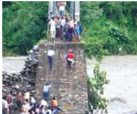
Fig. 8.25: Rescuers helping people cross a damaged bridge and road
