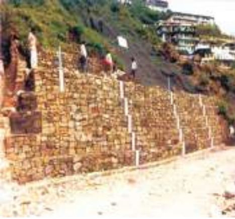
Fig. 7.25: Gabion wall made of boulders and wire baskets
