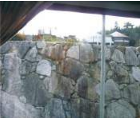
Fig. 7.29: Random Rubble Boulder Masonry Wall
