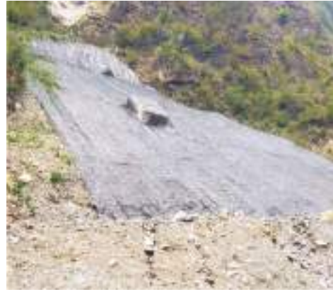
Fig. 7.44: Geosynthetic sheets used for stabilizing slopes
