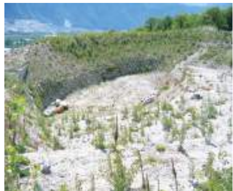
Fig. 7.40: Debris Catch Traps to avoid impact of debris flows
