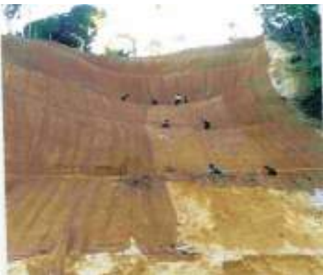
Fig. 7.5: Jute mats used for slope stabilization and vegetative growth
