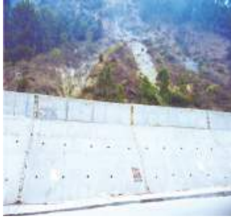
Fig. 7.20: Block masonry retaining wall with weep holes
