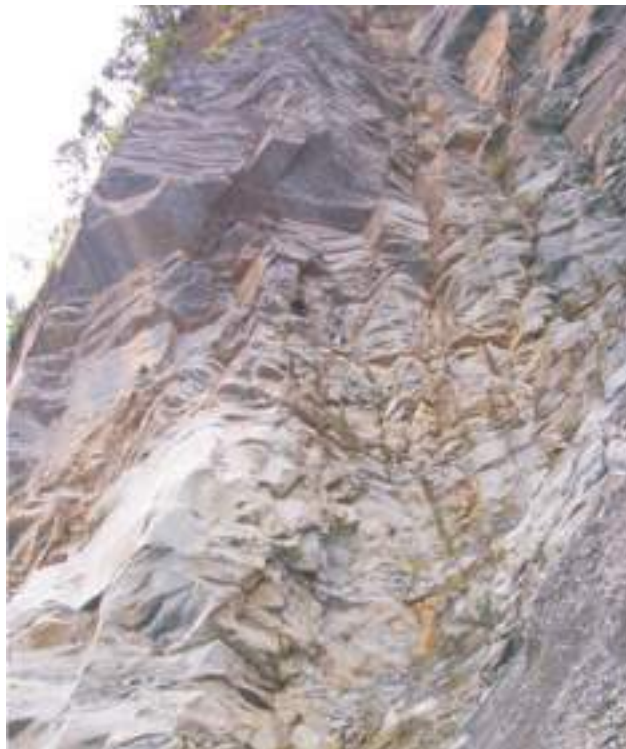
Fig. 1.6: Toppling Failure in Rocks
