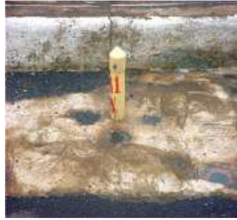
Fig. 6.2: Inclinometer installed to identify depth of slip surface
