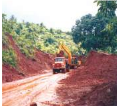
Fig. 8.11: JCB and Loader used in removing and disposing landslide debris
