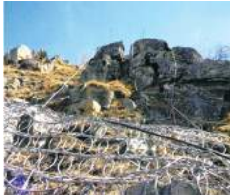
Fig. 7.46: Chain and cable type ring nets for preventing rock / boulder fall
