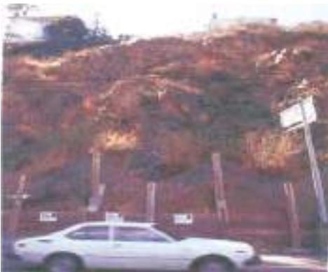
Fig. 7.41: Fencing with metallic nets and girdles for saving roads, vehicles and passerbyes from the landslides
