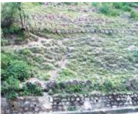
Fig. 7.47: Drum wall for mitigating landslide
