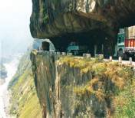
Fig. 8.8: Steep and negative slopes - a challenge to landslide managers
