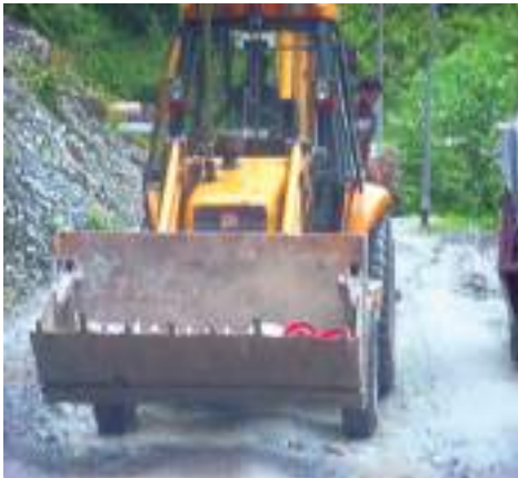
Fig. 8.10: Bull dozer for clearing road
