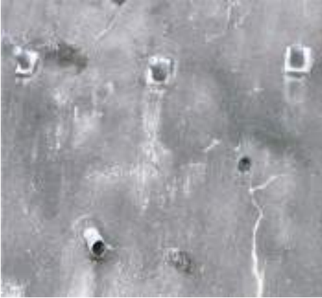
Fig. 7.31: Nailing for slope reinforcement
