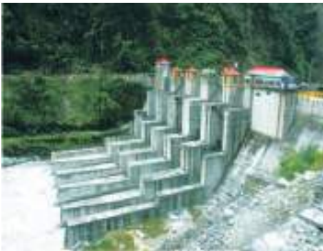
Fig. 1.22: Sudden and fast drawdown results in subsidence / landslides
