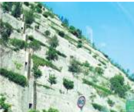
Fig. 7.59: Benching, retaining structures, drainage and plantation
