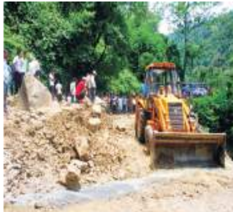
Fig. 8.17: Bulldozer clearing landslide debris from road side
