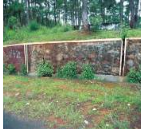
Fig. 7.26: Boulder masonry walls with joints to adjust minor deformations
