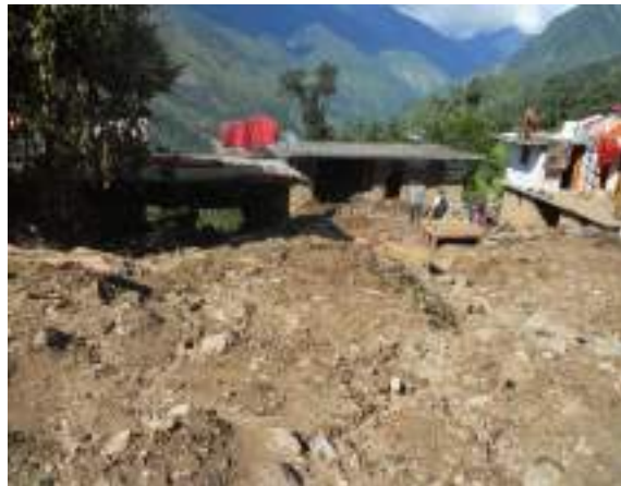
Fig. 27. View of the houses damaged by water saturated debris in Salami village.
