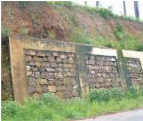
Fig. 7.27: Banded Random Boulder wall without masonry
