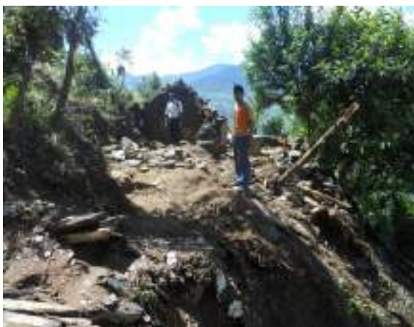
Fig. 24. View of the house ravaged by landslide.
