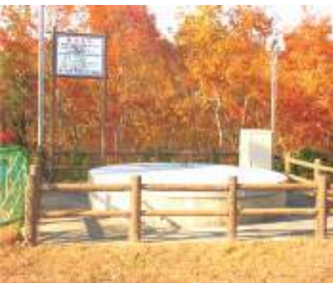
Fig. 7.11: Covered well for subsurface drainage
