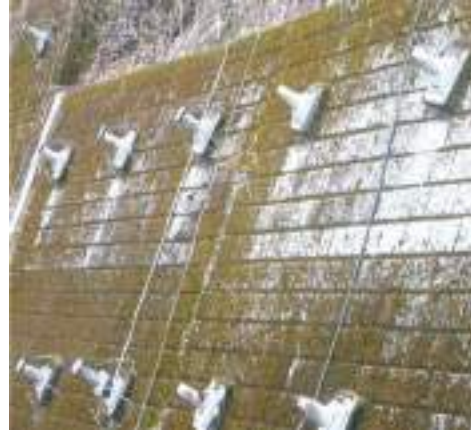
Fig. 7.32: Steel anchors and mesh used as preventive measure
