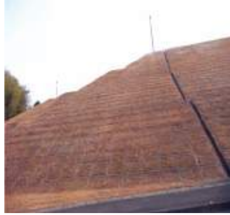
Fig. 7.14: Surface lined drains to dispose off water properly
