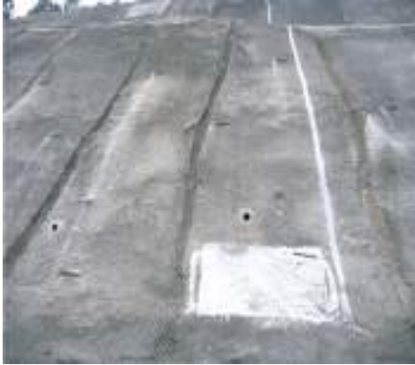
Fig. 7.43: Shotcreting with wire mesh and weep holes
