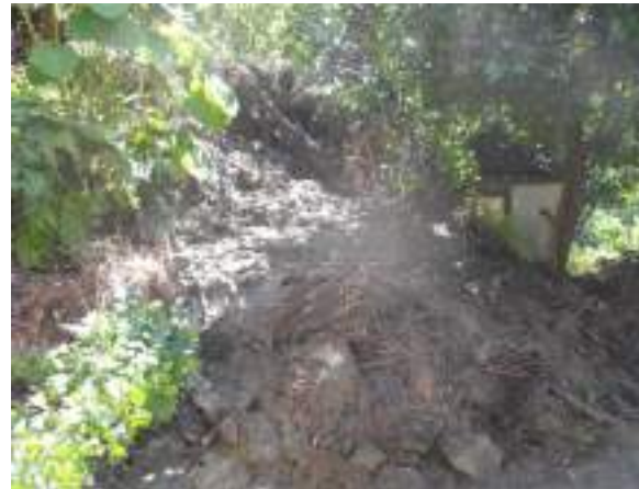
Fig. 42. View of debris overrunning a toilet at Bengar tok.
