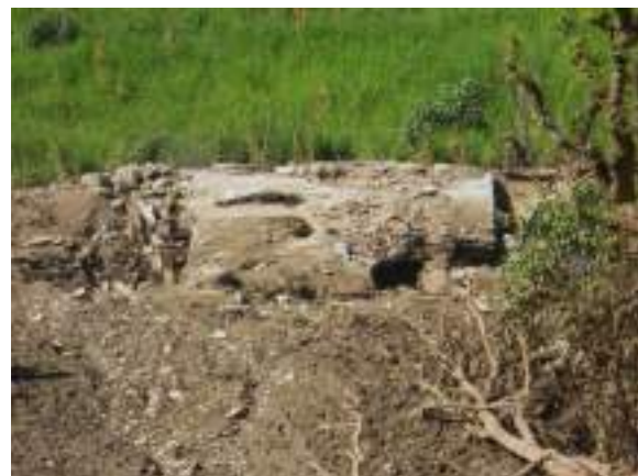
Fig. 40. View of completely damaged house at Kirora Malla.
