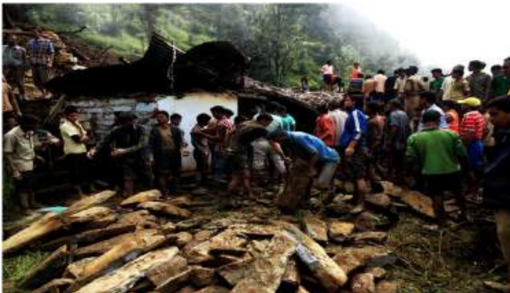
Fig. 38. Photograph showing devastation due to landslide in Kirora Malla.
