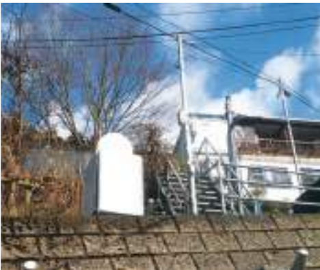
Fig. 6.5: Geodetic surveying for studying spatial movements in slopes
