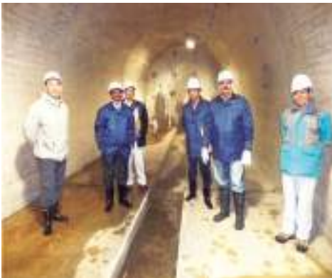
Fig. 7.9: Drainage Gallery / Tunnels to collect and dispose off subsurface water
