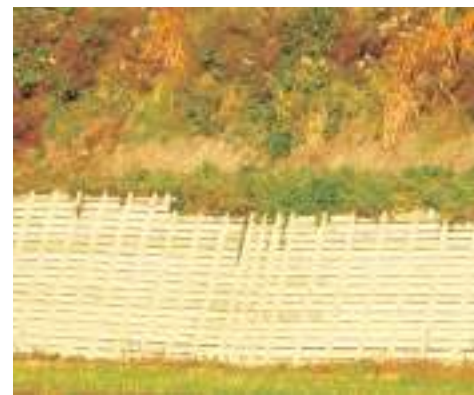
Fig. 7.18 Timber stitching for preventing slope failure
