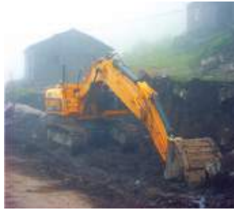
Fig. 8.9: JCB clearing debris
