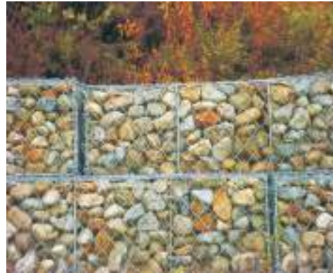
Fig. 7.28: Random Boulder Gabion Wall with wire crates
