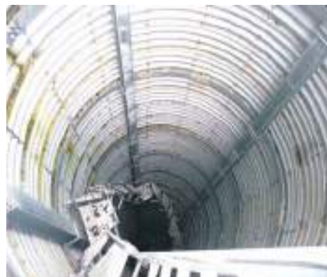
Fig. 7.12: Open well for collecting subsurface water from landslide site
