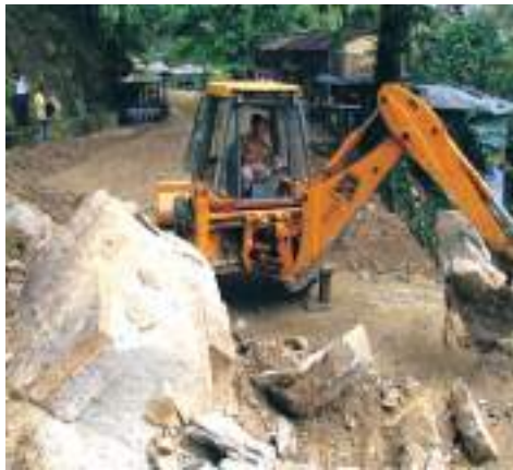
Fig. 8.16: Mechanical breaking and removal of big boulders
