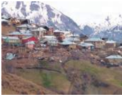
Fig. 1.47: Earthquake induced landslide causing damages to a cluster of houses
