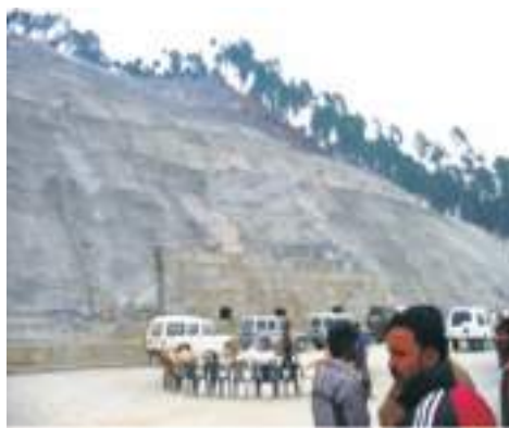
Fig. 7.22: Multiple remedial measures for stabilizing landslide site
