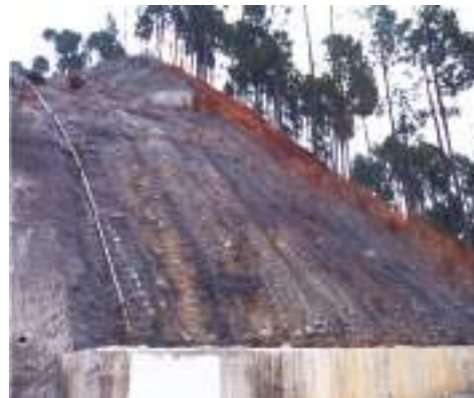
Fig. 7.6: Slope protection with geogrid helps prevent surficial rock failures
