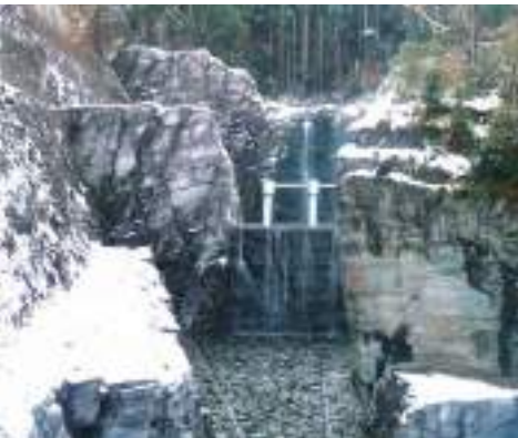
Fig. 7.17: Debris Control Structures and Mechanism
