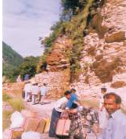
Fig. 1.5: Field photo showing topple failure
