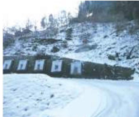
Fig. 7.36: Rock bolting for slope reinforcement
