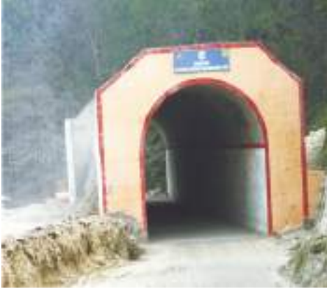
Fig. 7.37: Tunnel to avert recurring and chronic landslide
