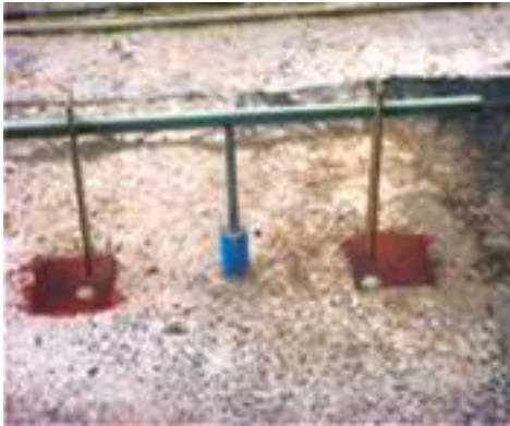
Fig. 6.3: Differential settlement Gauge for monitoring vertical movement
