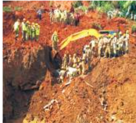
Fig. 8.5: Fire Gaurds and Civil Defence personnel extricating a dead body
