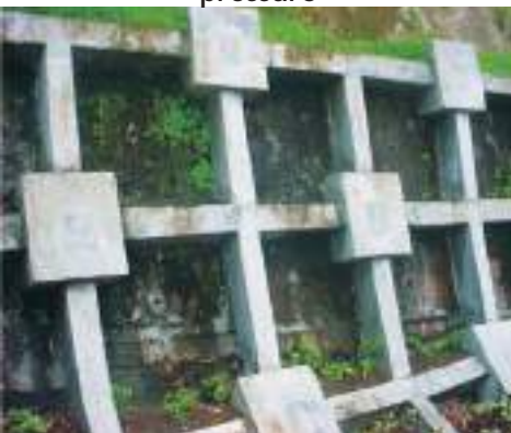
Fig. 7.35: Rock anchors with tie beams made of reinforced concrete
