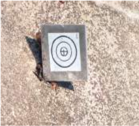
Fig. 6.13: Reflecting stickers used to monitor surficial slope displacements
