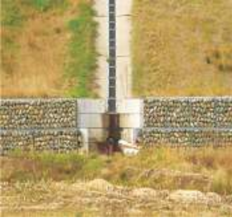
Fig. 7.13: Boulder Gabion wall with surficial drainage system
