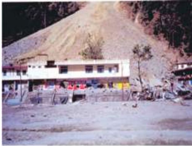
Fig. 1.62: Landslide buries both commercial and residential buildings besides blocking the highway
