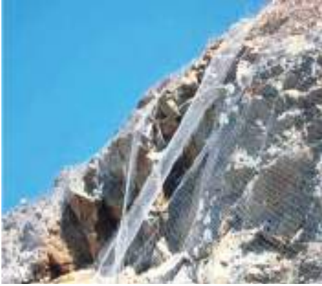
Fig. 7.49: Catch nets for restraining rock fall
