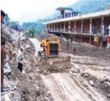
Fig. 8.4: Bull dozer clearing landslide debris from the road
