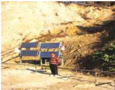
Fig. 6.15: Solar panels used for power supply in automated monitoring system
