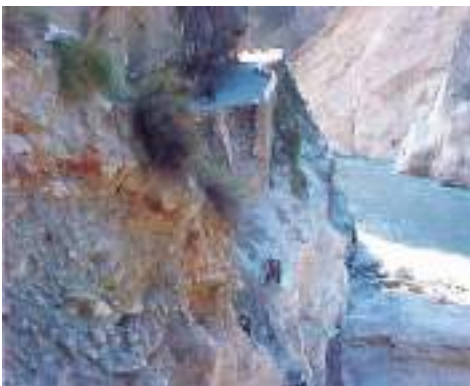
Fig. 8.24: Road washed off by landslide makes access difficult for rescue & relief
