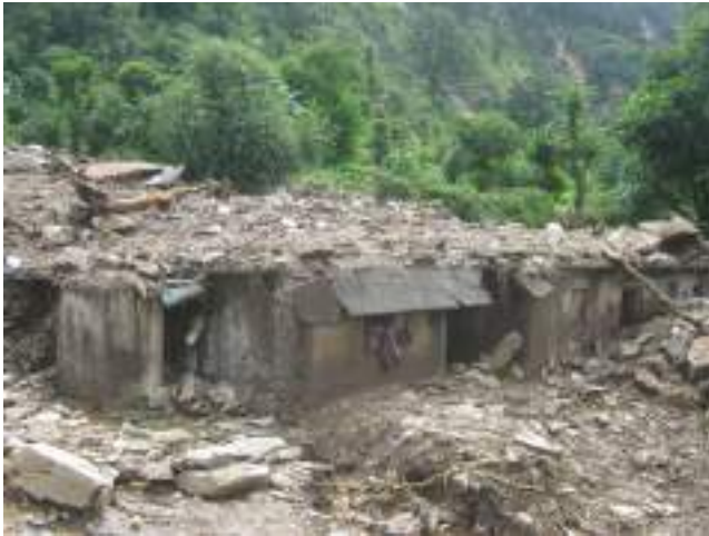
Fig. 10. Damaged houses in Mangoli village.
