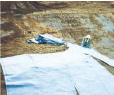
Fig. 7.3: Application of Geosynthetic mats for slope stability
