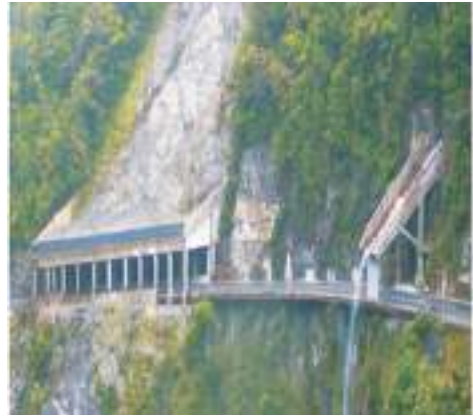
Fig. 7.50: An open rock shed
