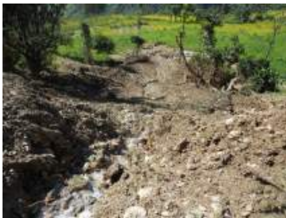
Fig. 39. Photograph showing debris flow at Kirora Malla.
